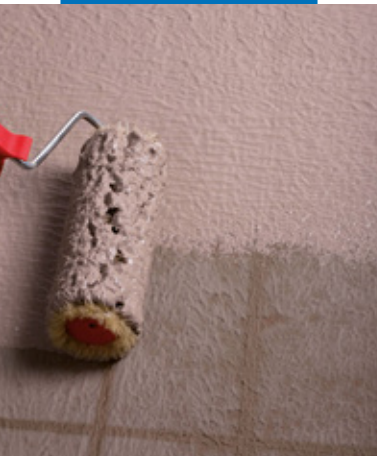
Waterproofing of details by roller
