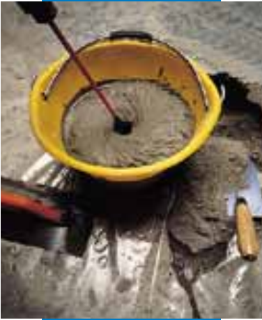
Nivorapid mixed with mechanical mixer
