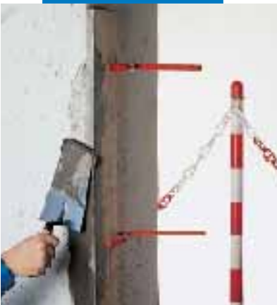
Repairing vertical arrise with Nivorapid
