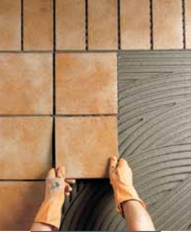
External installation of klinker tiles
