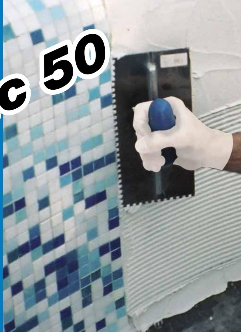
**Isolastic 50** is a latex to be mixed with **Kerabond T**, **Kerafloor** and **Adesilex P10** to improve their performances and deformability to meet the requirements of class C2 (improved cementitious adhesive) according to EN 12004 and those of class S1 according to EN 12002.
