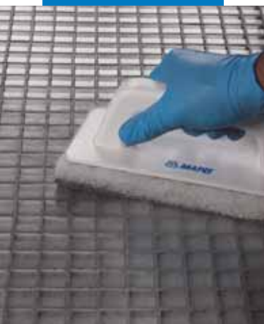
Cleaning with a Scotch-Brite® pad
