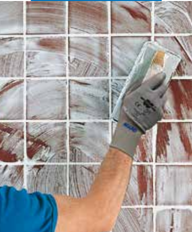
Laying the product with a rubber float
