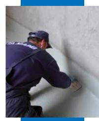
Mapelastic Foundation spread on by trowel to waterproof against water in negative pressure
