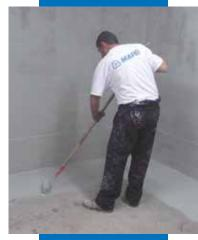
Mapelastic Foundation spread on by roller to waterproof against water in negative pressure
