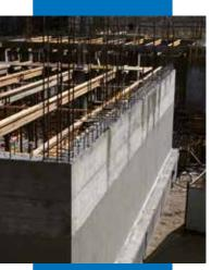
Retaining wall waterproofed after casting using Mapelastic Foundation
